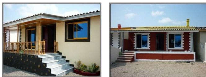
Figure 2: Veranda in South Axis of Building
